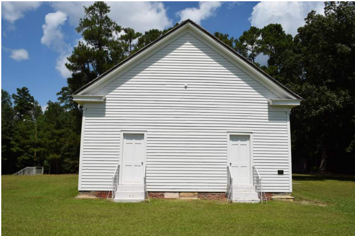
Figure 6: Facade (south elevation) of church, view to the north
