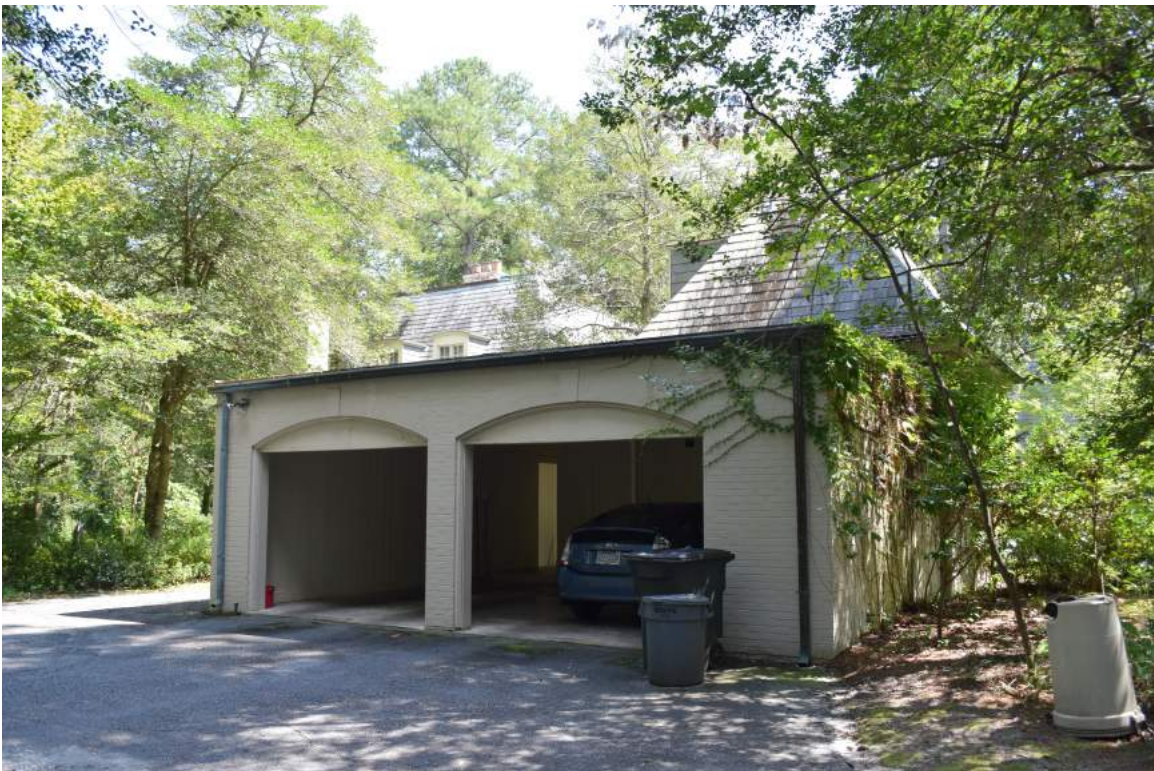
Figure 22: Ficklen House attached garage on north elevation, view to the south-southeast
