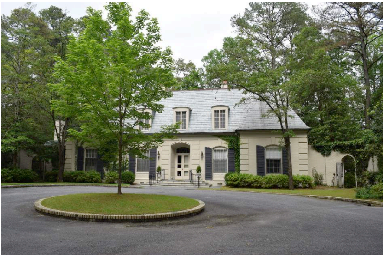
Figure 20: Ficklen House facade and driveway, view to the east-northeast
